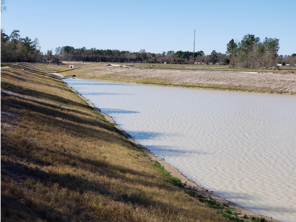
Portions of Detention Pond #1 Are Stabilized
