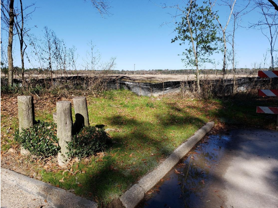
Grass Stabilization is Well Established on Village Springs Drive
