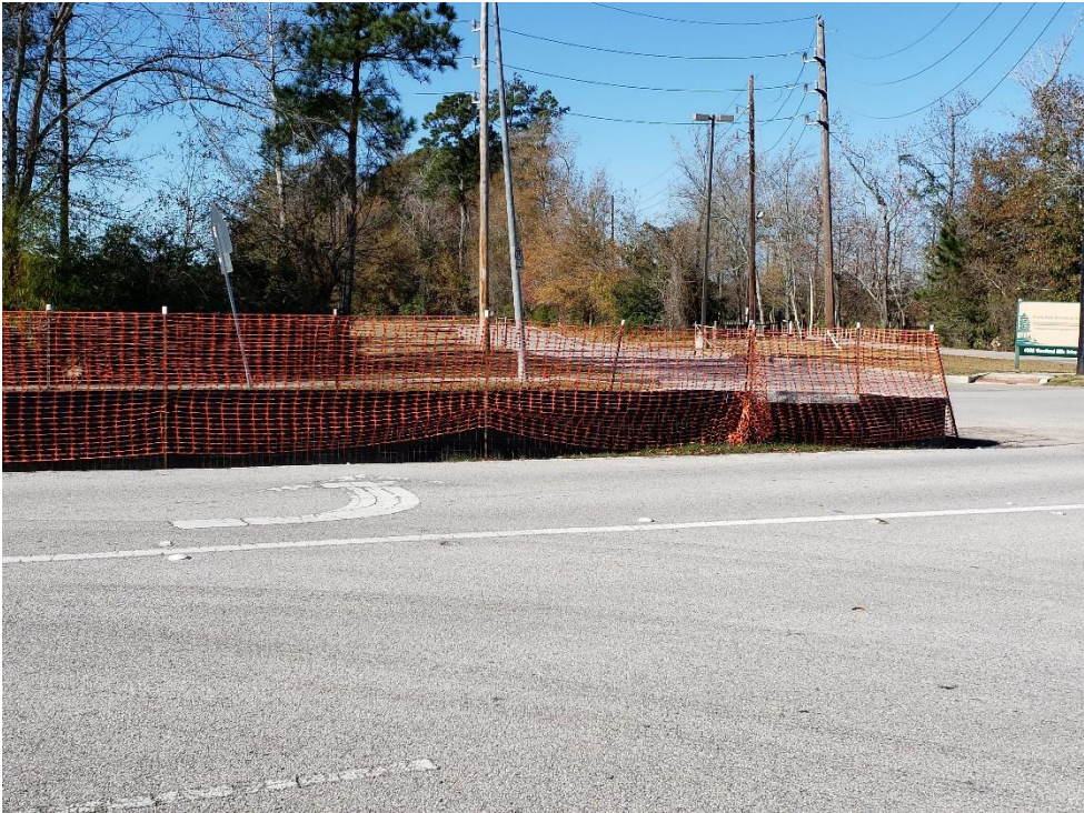
Median Protection on Woodland Hills Drive
