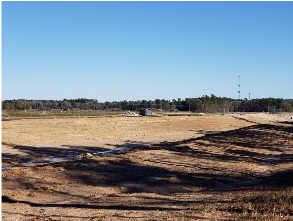
View of Detention Pond #2 Looking Northeast Note: Detention pond has not been stabilized
