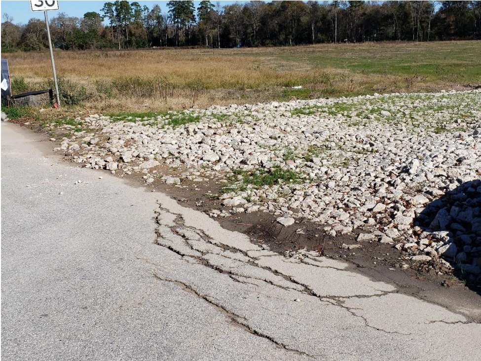
View of Construction Site Entrance on Woodland Hills Drive Note: Light tracking
