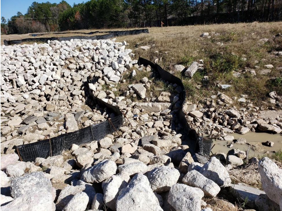
View of Outfall of Detention Pond #1 to Taylor Gulley Note: Silt fences are well maintained
