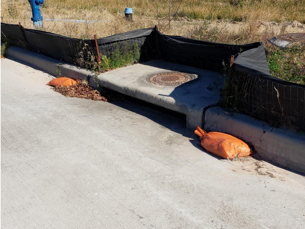
Inlet Protection on Woodland Hills Drive
