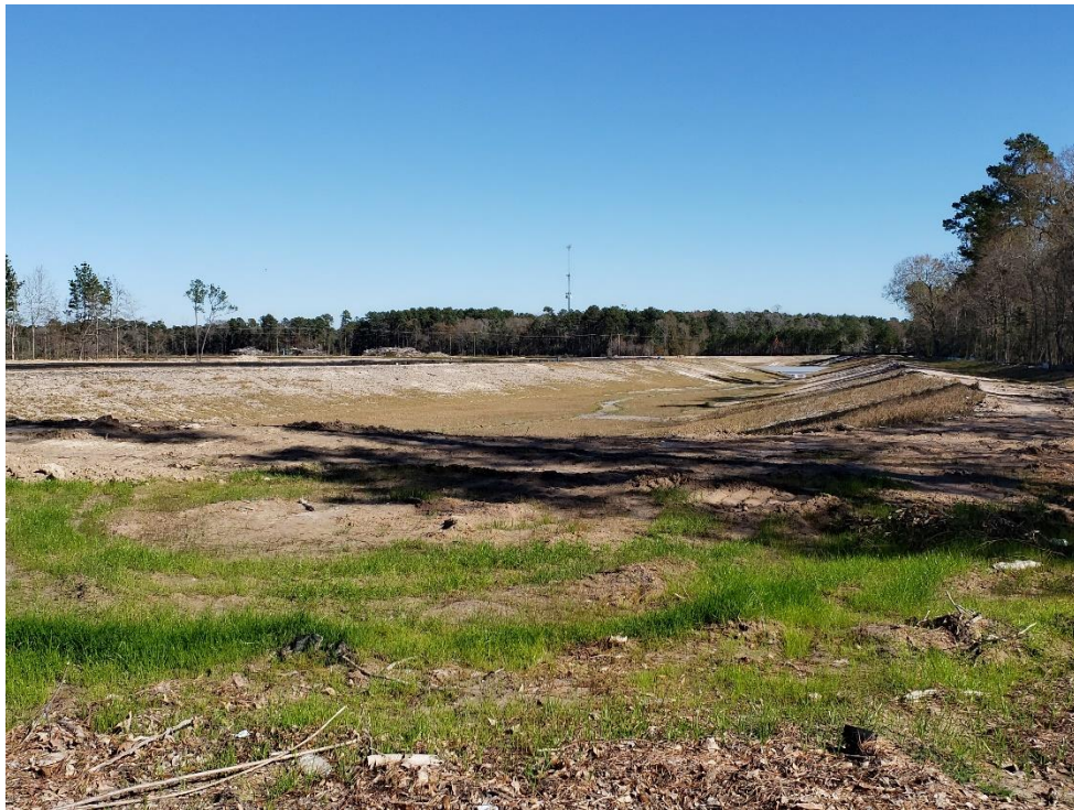
View of Detention Pond #1 Looking East
