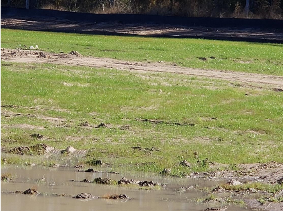
View of South Construction Area with Grass Stabilization
