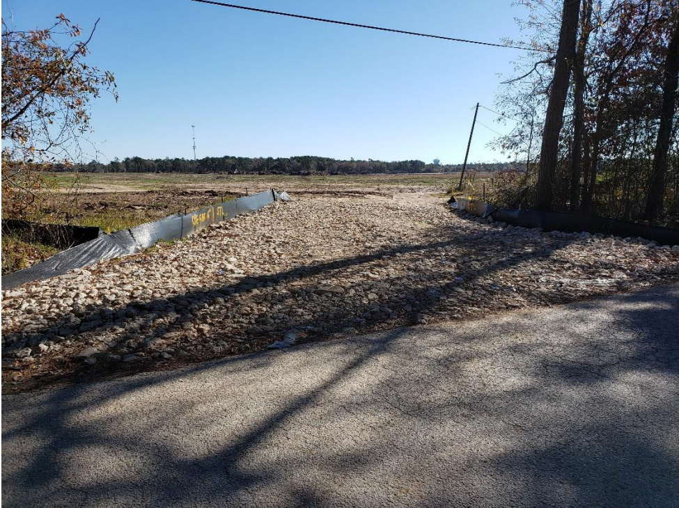
View of Construction Entrance on Webb Road
