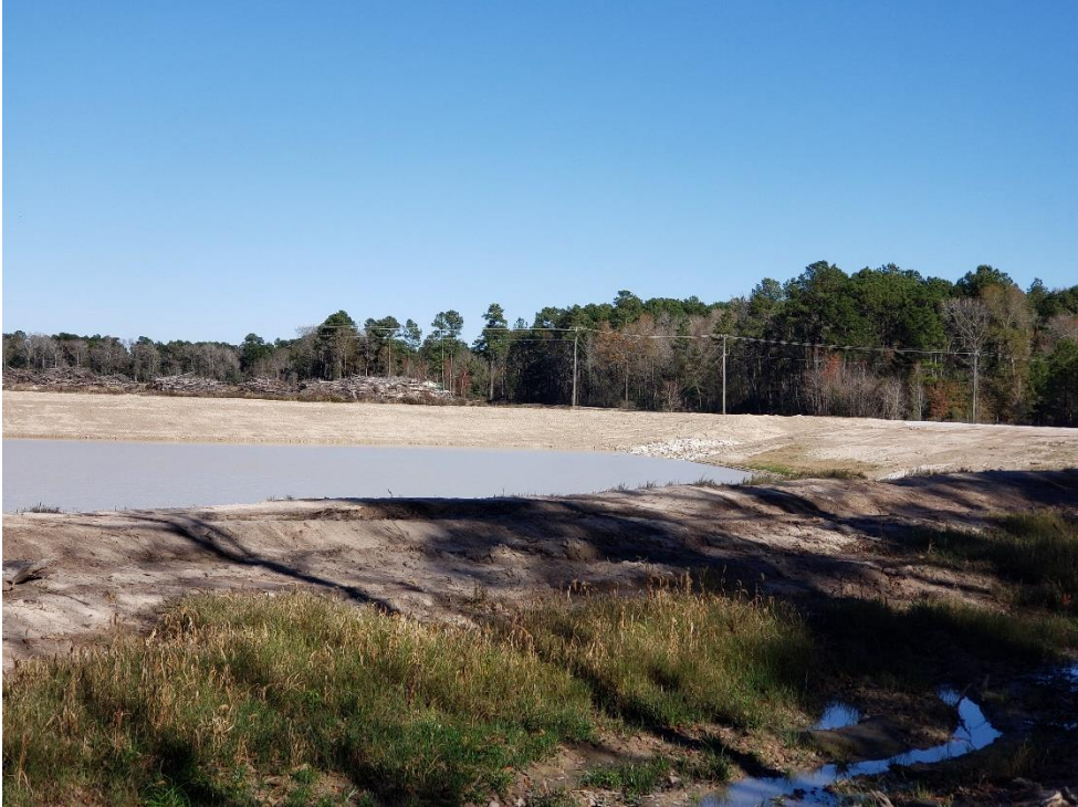
View of Detention Pond #1 Looking Northeast Note: Pond is partially stabilized
