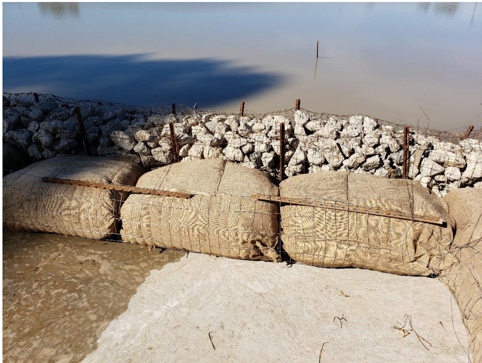
Close View of Hay Bales Secured to Gabions
