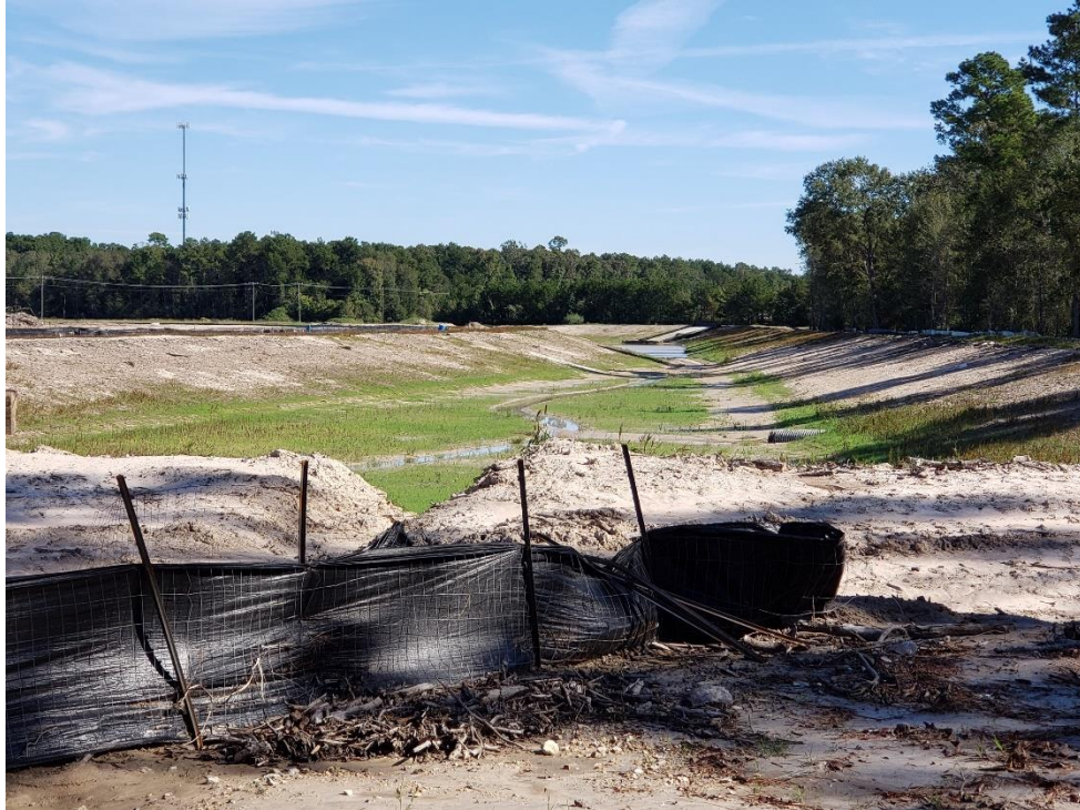
View of Detention Pond #1 Looking East Note: Partial stabilization in bottom of pond
