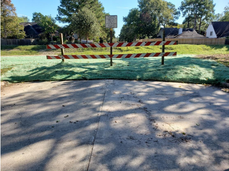
View of Creek Manor Drive with Curlex Blanket Stabilization
