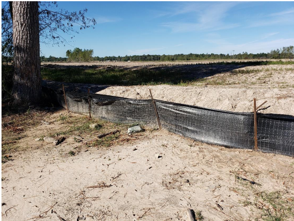
Repaired and Maintained Silt Fencing
