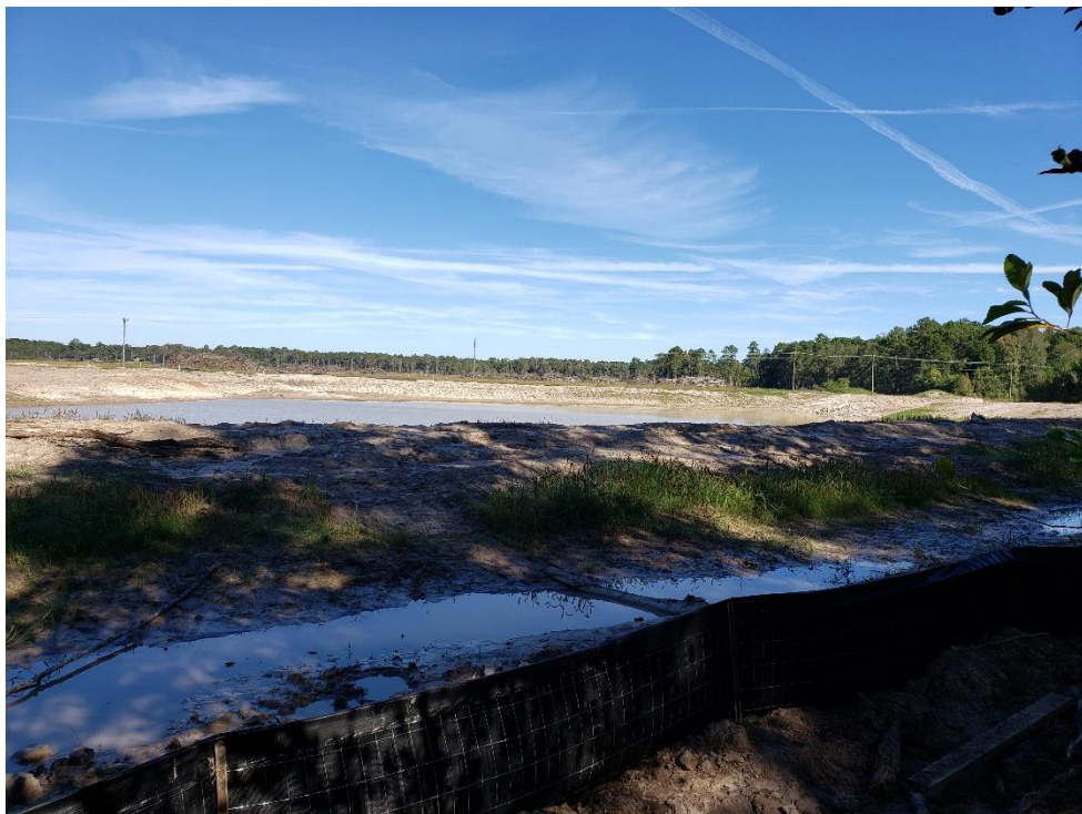
View of Detention Pond #1 Looking Northeast
