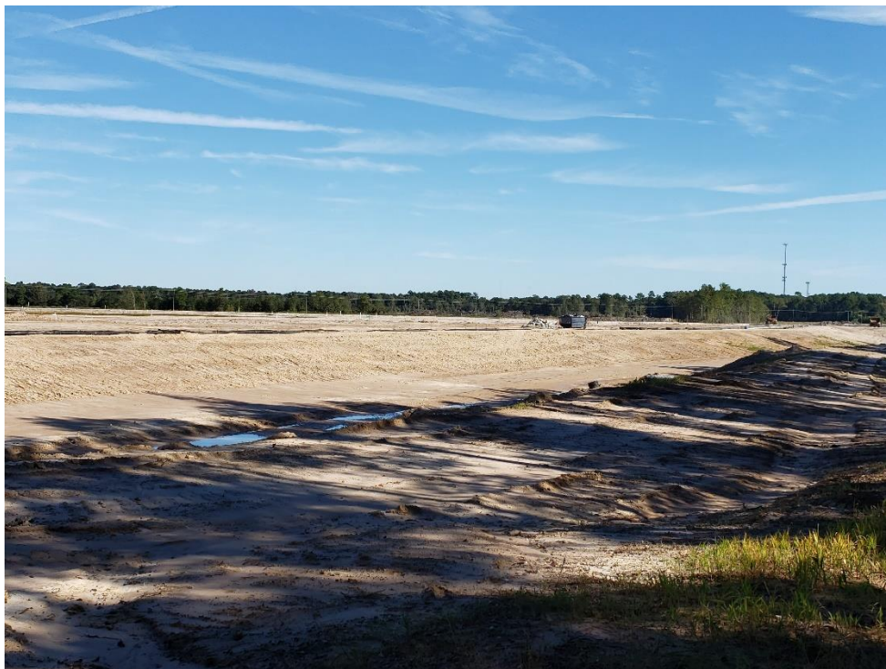
View of Detention Pond #2 Looking Northeast
