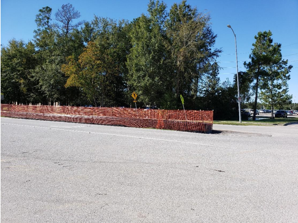
Median Protection on Woodland Hills Drive
