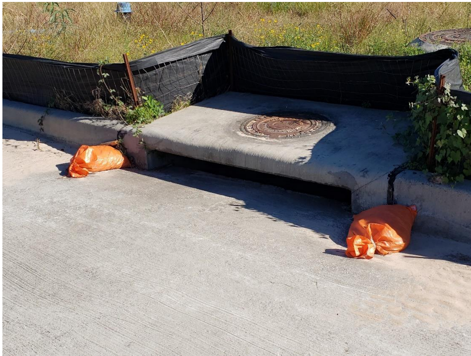
Inlet Protection on Woodland Hills Drive Note: Small amount of silt accumulation
