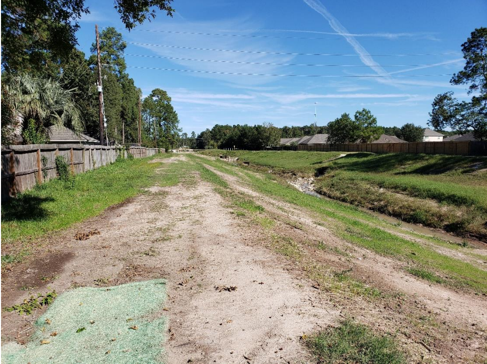
View Looking North along Taylor Gulley
