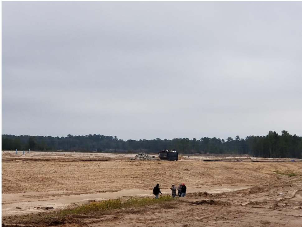
Construction Activity Taking Place on Detention Pond #2
