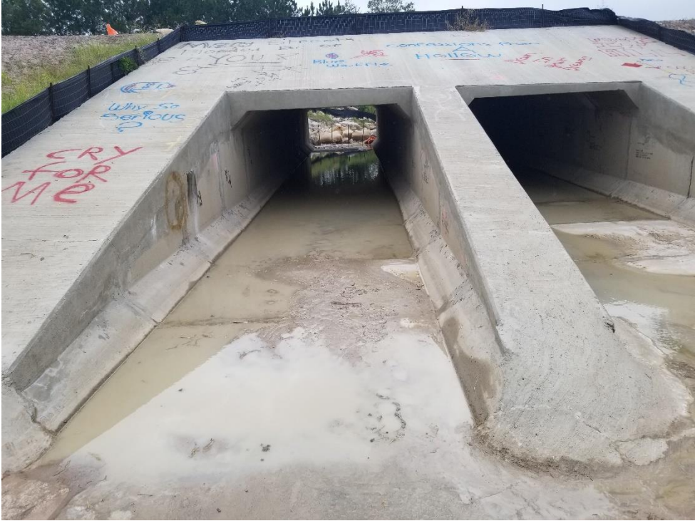
Sediment Removed from Outfall Structure
