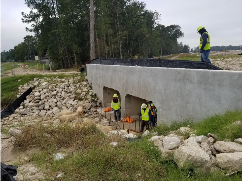
Installing Hay Bales at Outfall Structure
