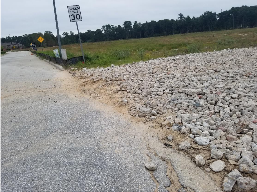
Construction Site Entrance on Woodland Hills Drive
