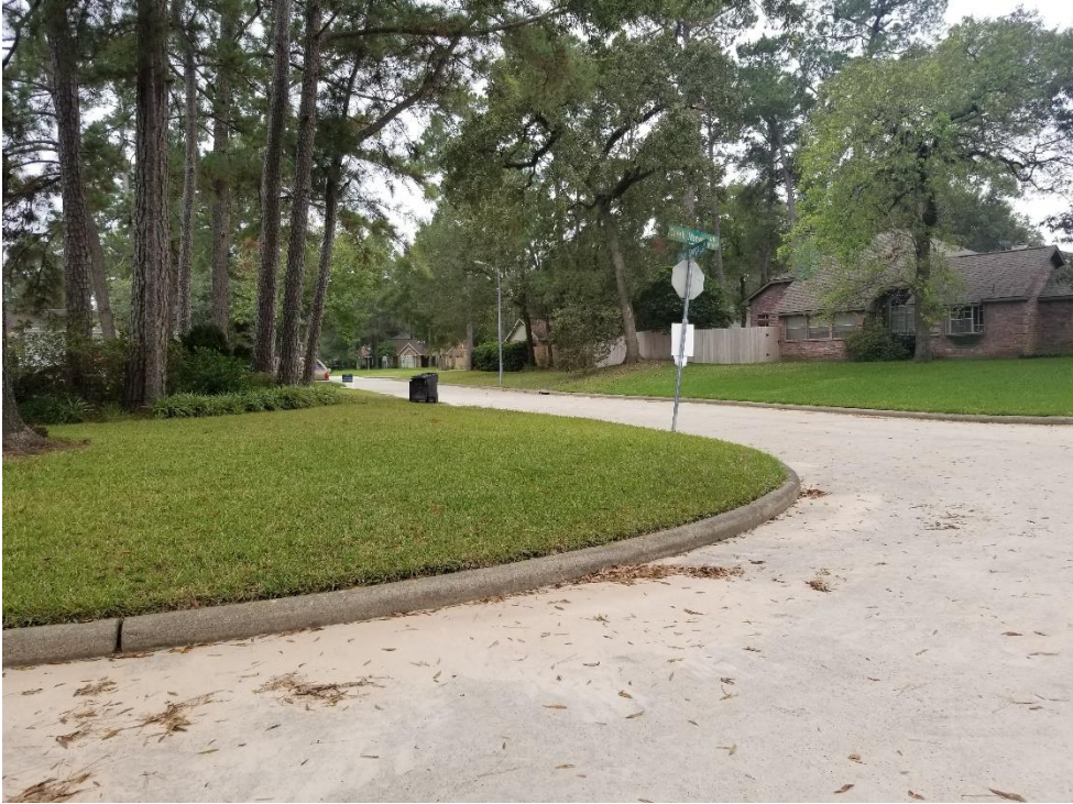
Creek Manor Drive Requires Sediment Removal
