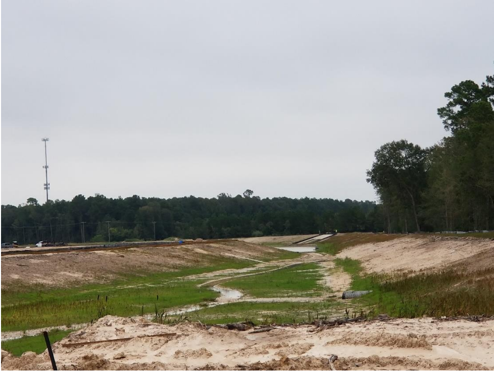
View of Detention Pond #1
