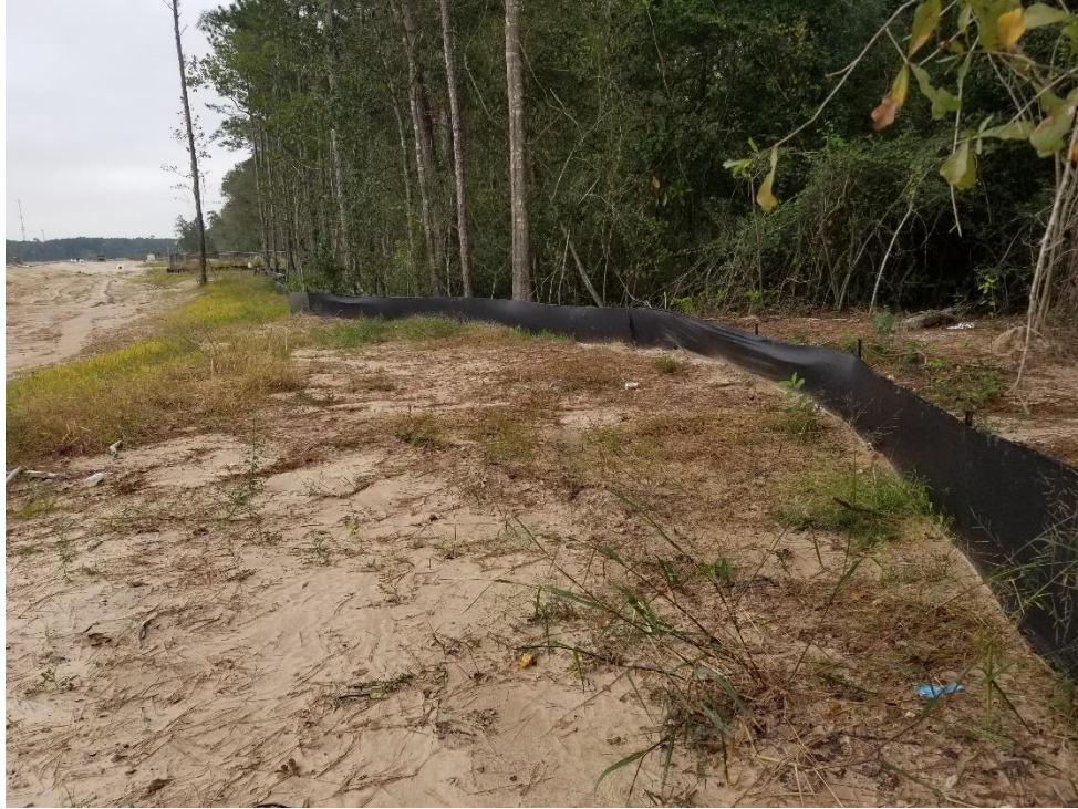
Silt Fencing in Good Shape
