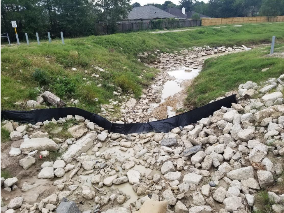
Newly Installed Silt Fence Across Taylor Gulley
