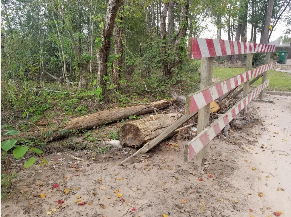
End of Village Springs Drive Requires Debris Removal
