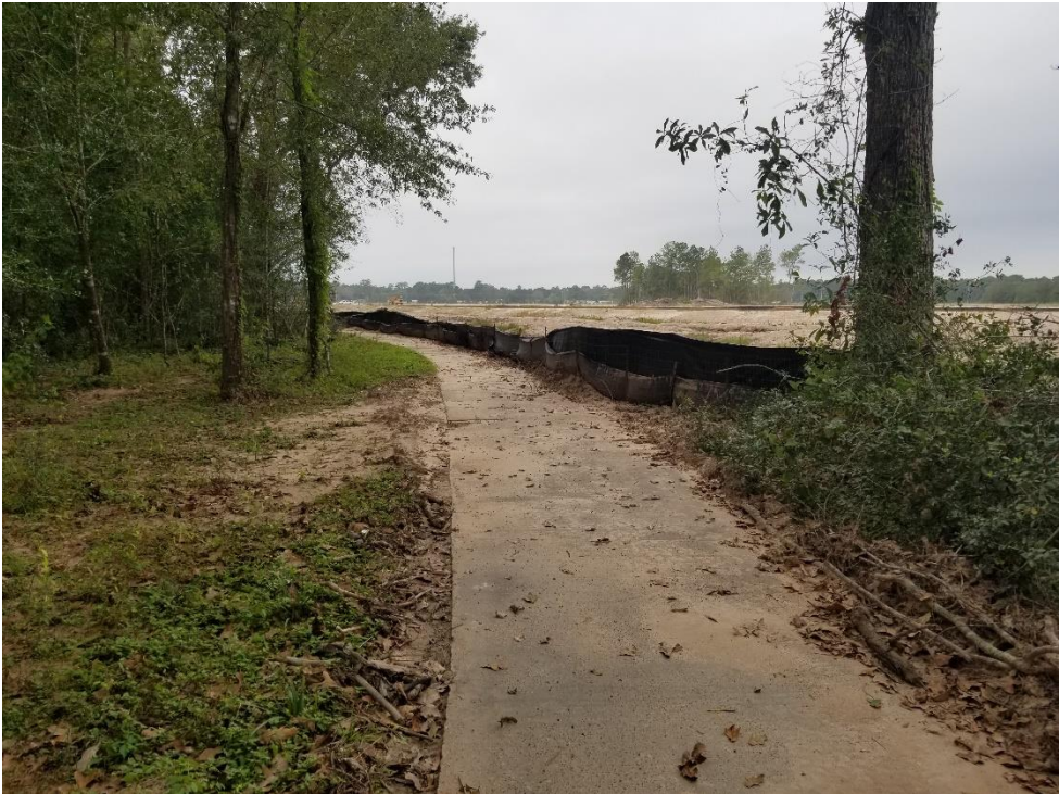
Newly Installed Silt Fence
