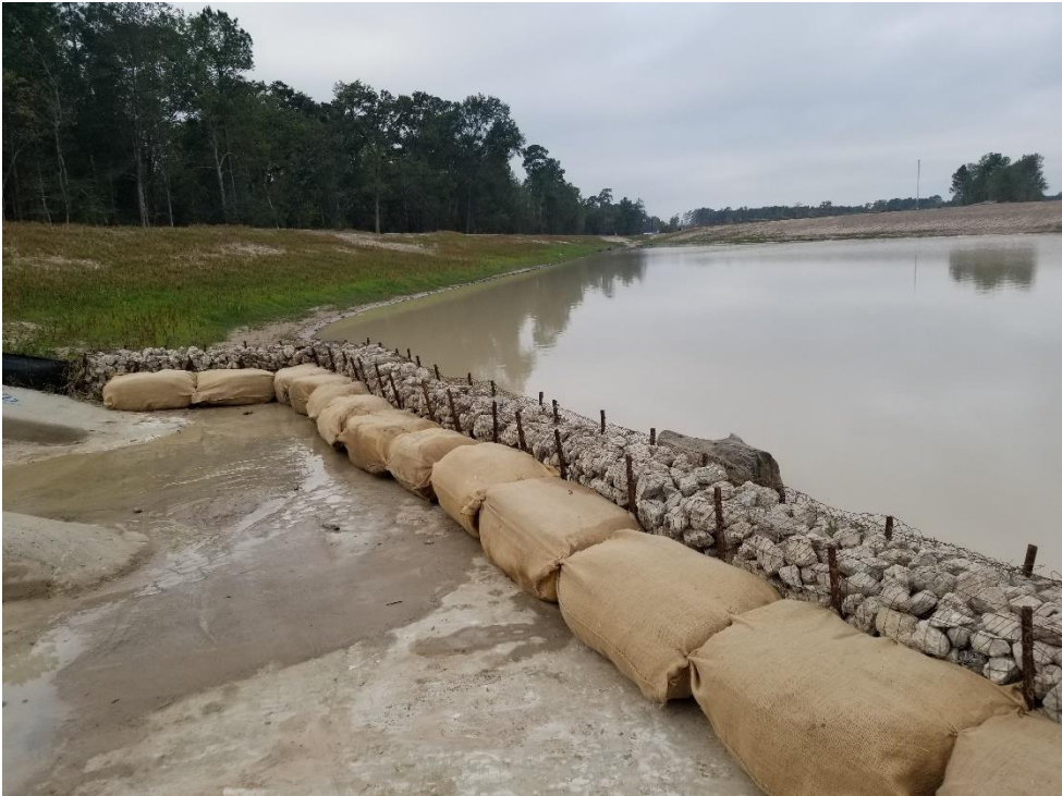
Hay Bales Have Been Installed at Intake of Outfall Structure
