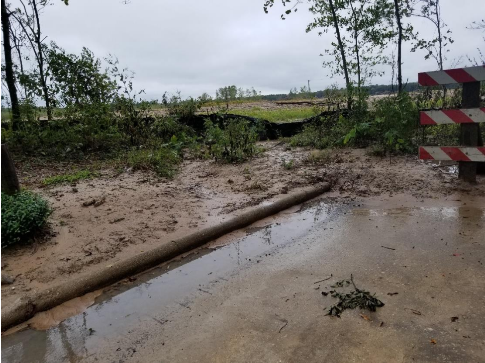
Remove Sediment and Stabilize Disturbed Area on Village Springs Drive
