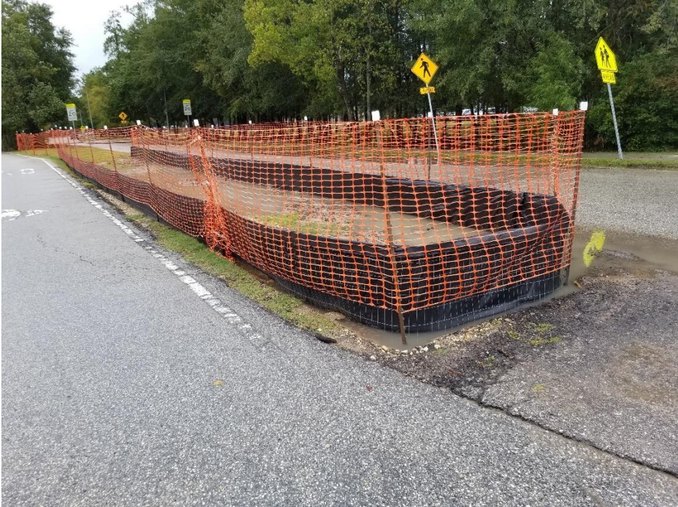
Median Protection on Woodland Hills Drive
