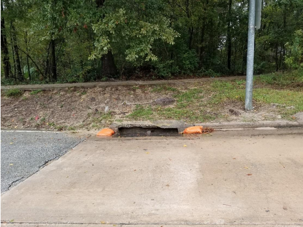
Clean Storm Sewer Inlet on Woodland Hills Drive
