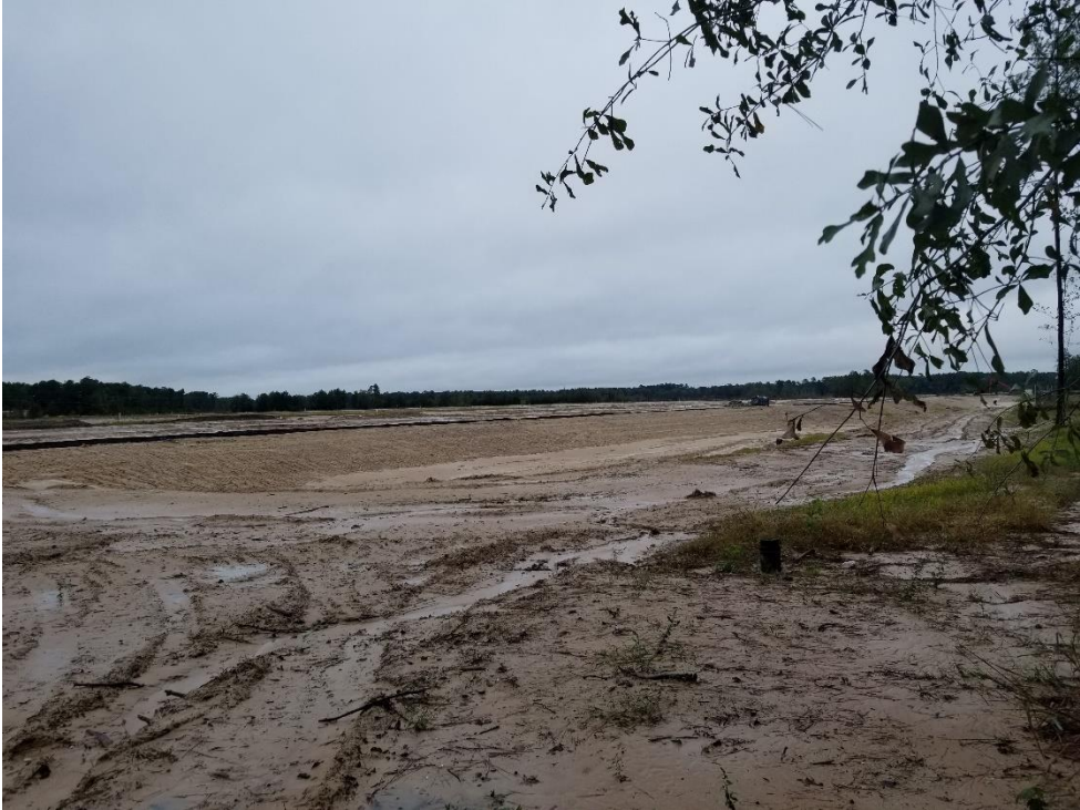
View of Detention Pond #2 Looking Northeast
