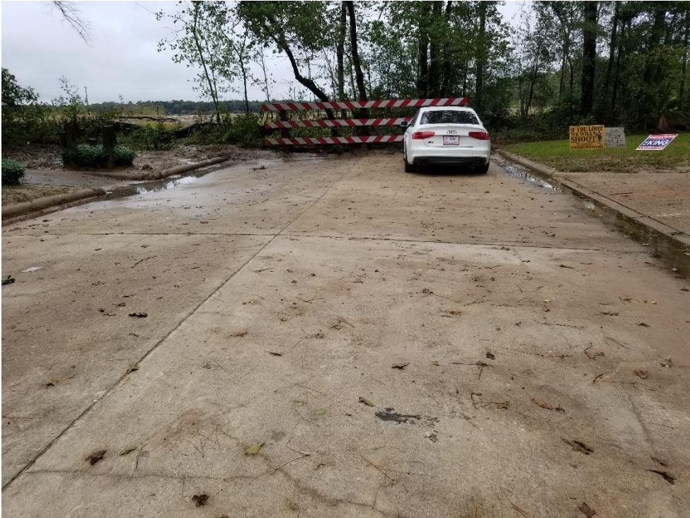
Village Springs Drive with Light Sediment
