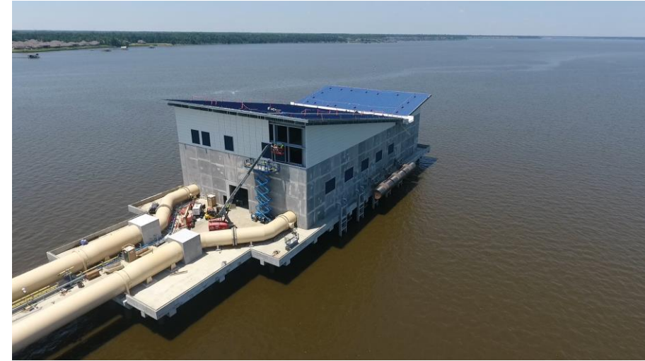
Influent Pump Station on Lake Houston
