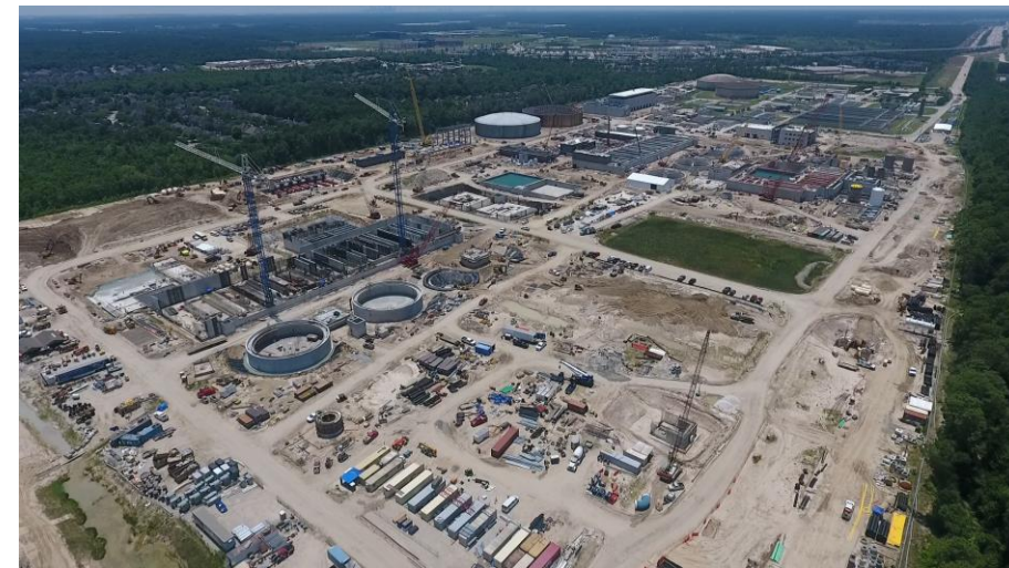
Northeast Water Purification Plant Expansion
