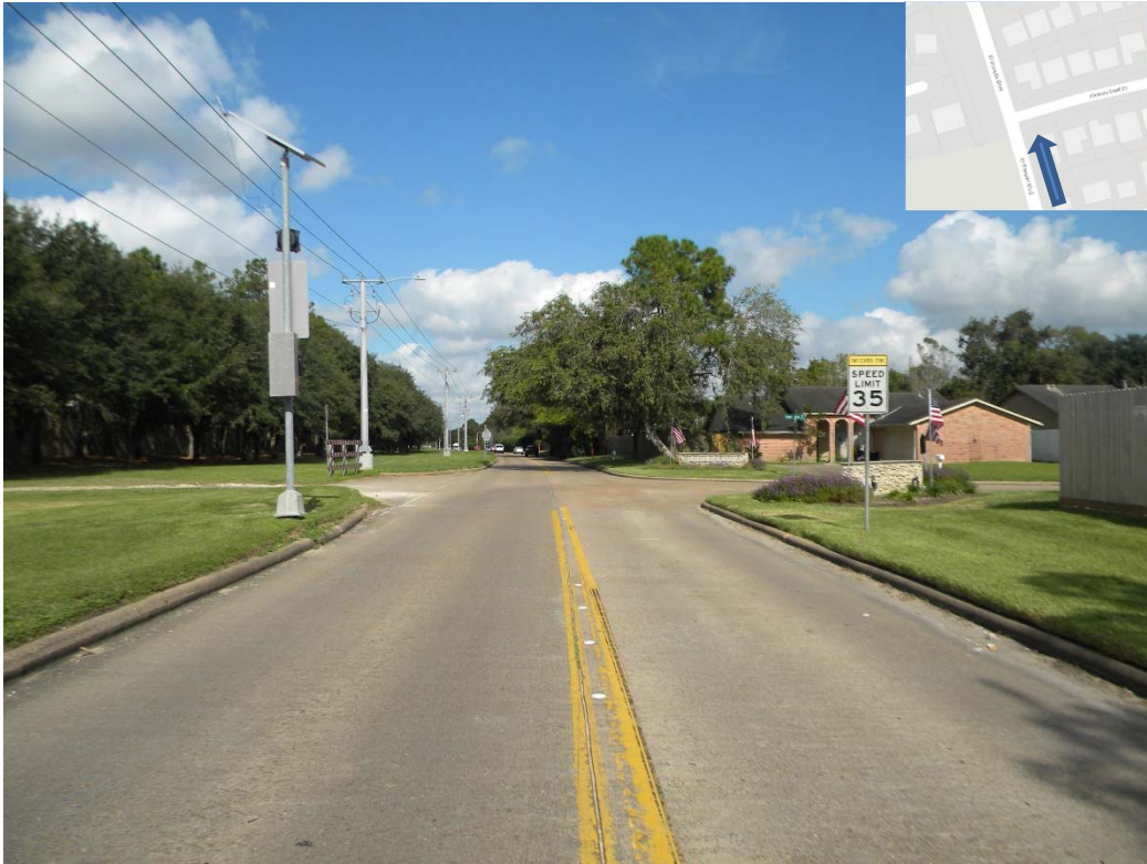
Facing North on El Dorado Boulevard – South of Hickory Knoll Drive
