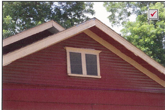
Original window in gable
