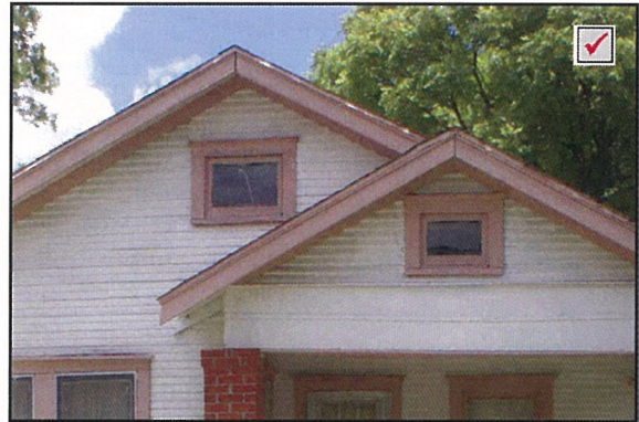
Original windows in gables
