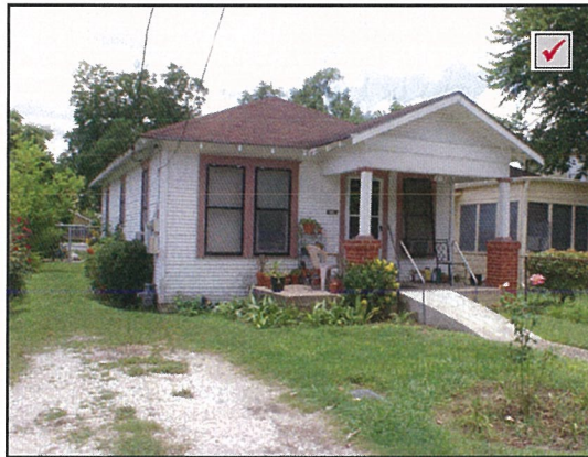
Concrete ramp to front porch, with handrails
