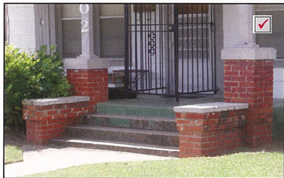
Brick porch column/base
