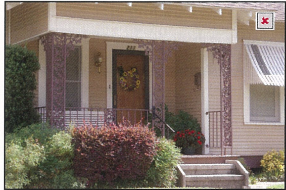
Incompatible ornamental metal replacement posts on a Craftsman house; these would be compatible with a Minimal Traditional house
