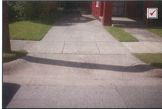
Poured concrete driveway
