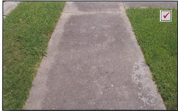
Poured concrete sidewalk
