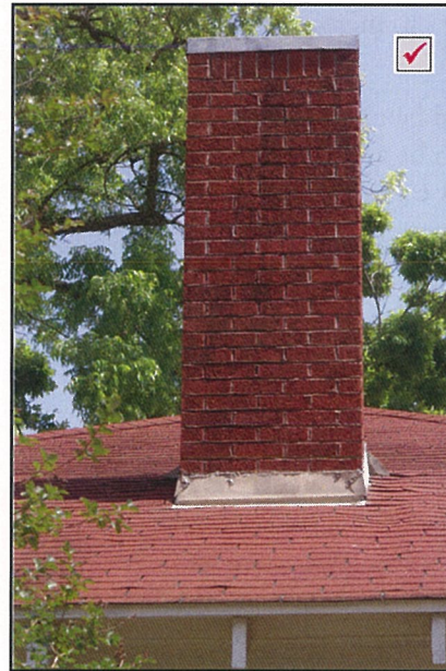
Chimney located on an interior wall
