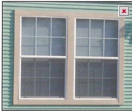
Six-over-six window (not original) with interior muntins
