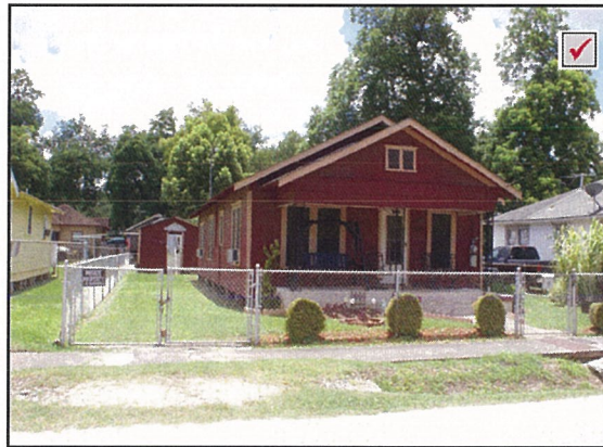
Typical gabled roof
