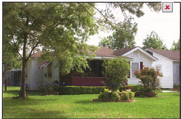
Incompatible screened-in porch
