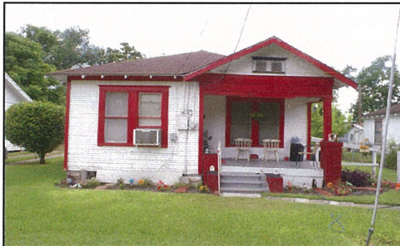
Hipped roof with front gable
