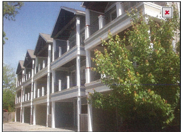
Streetscape in neighborhood of high density townhouses
