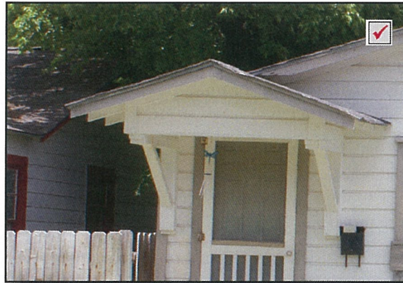
Pent roof over front door
