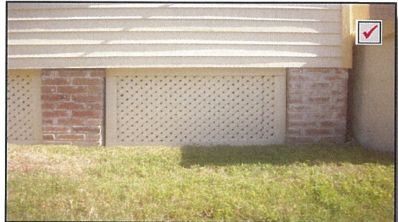
Lattice panel, framed between piers
