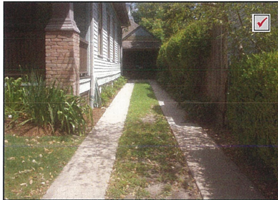
Poured concrete driveway strips
