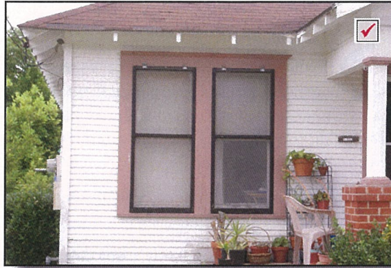
One-over-one original window with exterior storm windows
