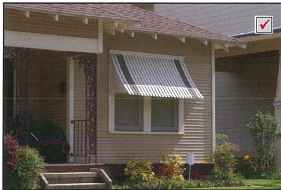
Metal awning over window
