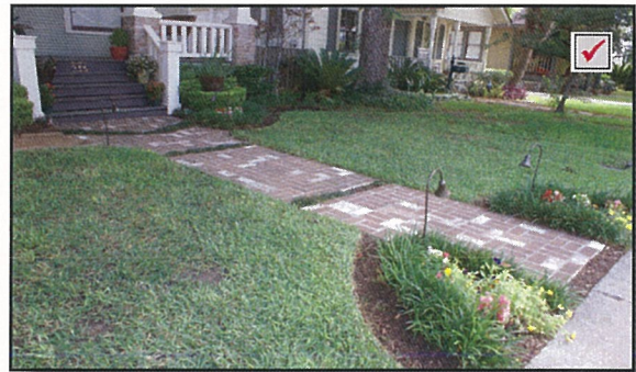
Walkway constructed of brick pavers
