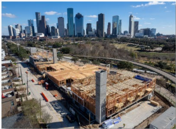
*2100 Memorial Construction Progress (January 2023)
