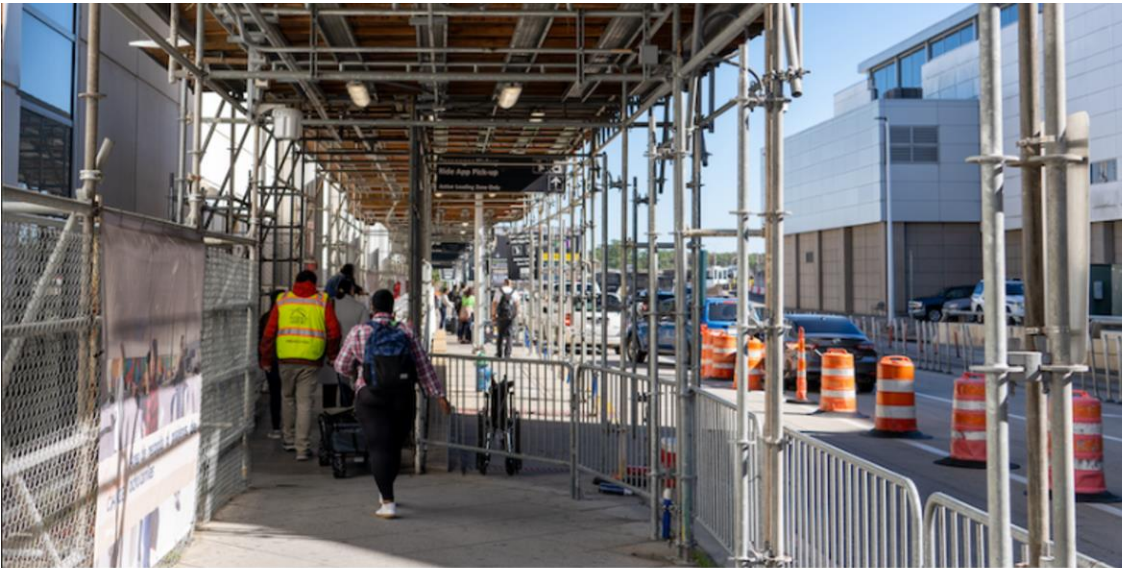
JANUARY 2022 TO DECEMBER 2024 Temporary Terminal E Arrivals Curb 1 Dedicated Lane
