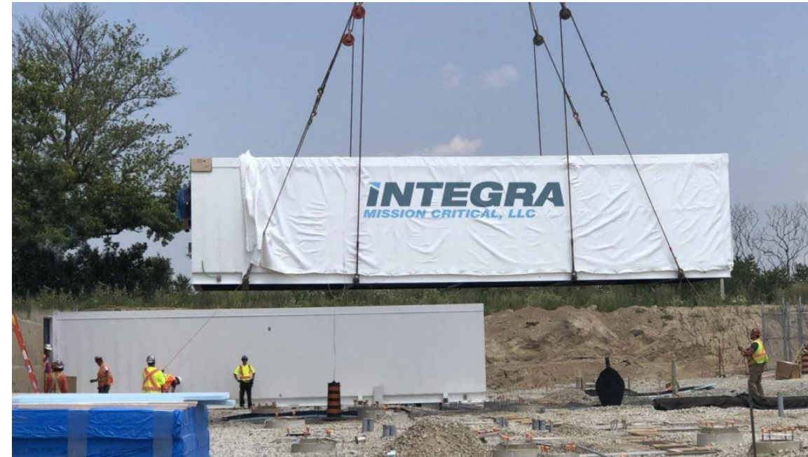
PowerBlox units are modular power rooms that offer climate-controlled protection for infrastructure housed outside a free-standing data center
