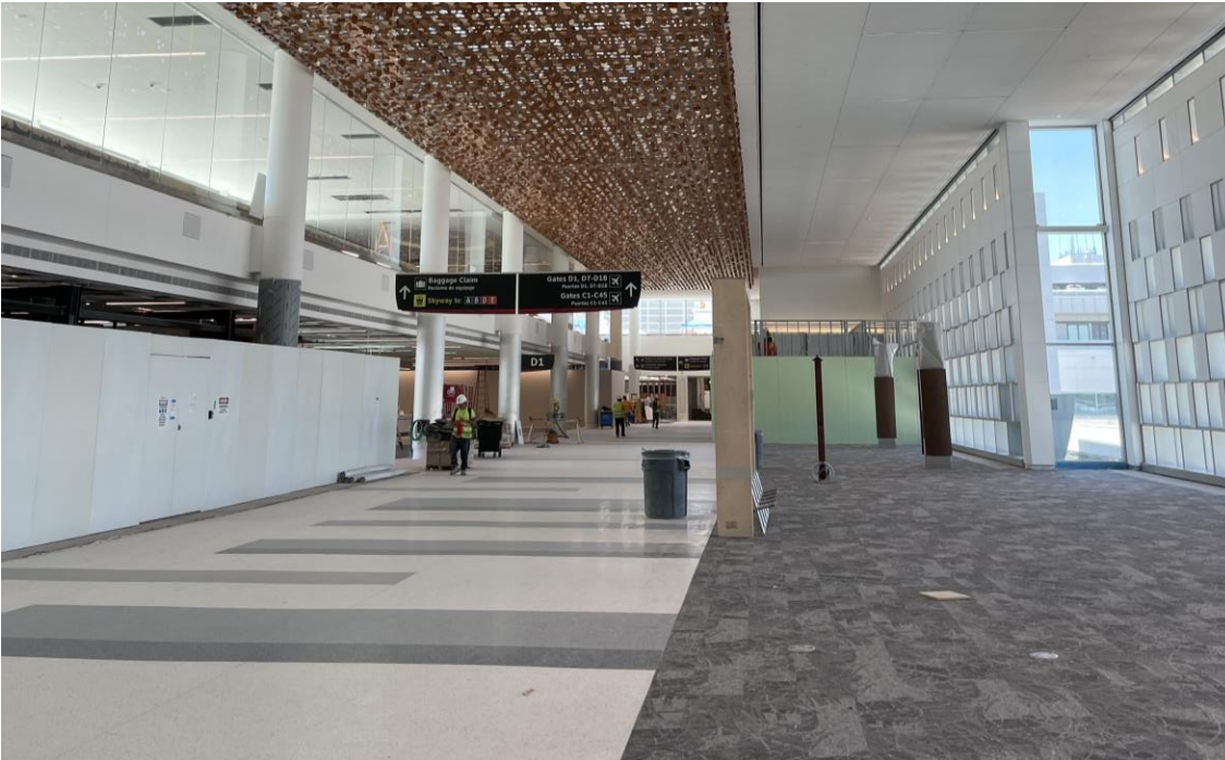
Carpeting, Wayfinding Signs Installed
