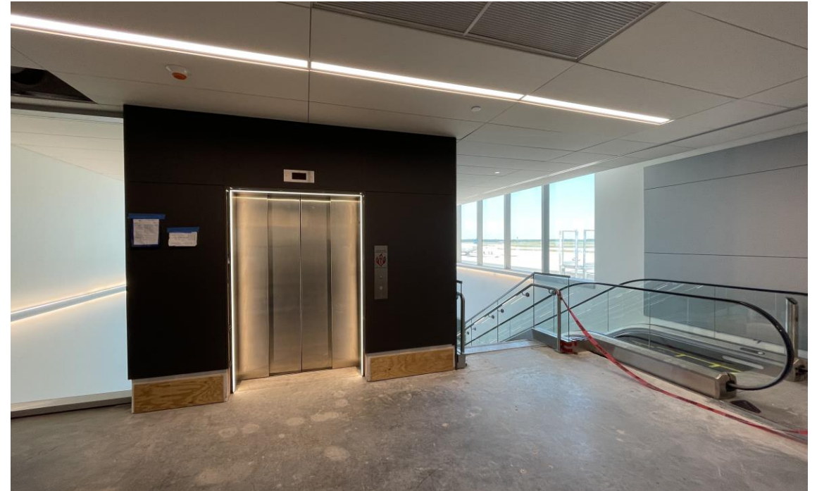
Elevator, Escalator, Stairs Installed
