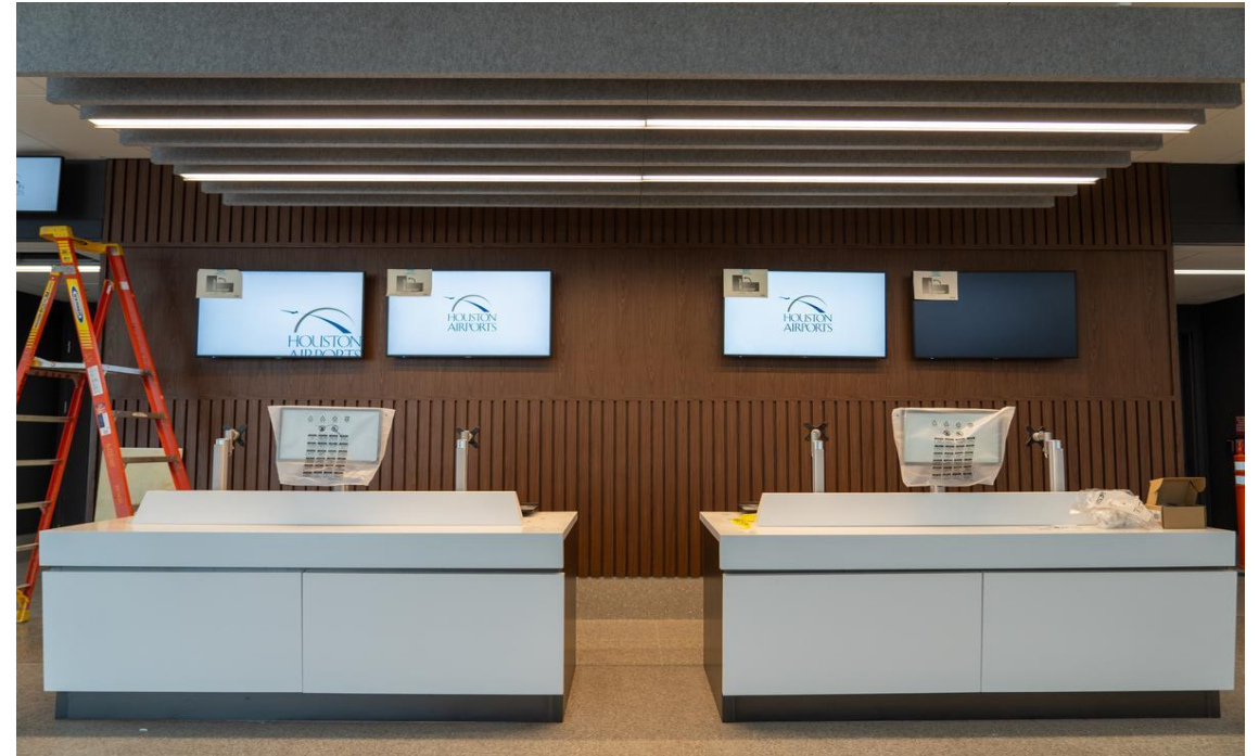
Customer Service Counters Installed
